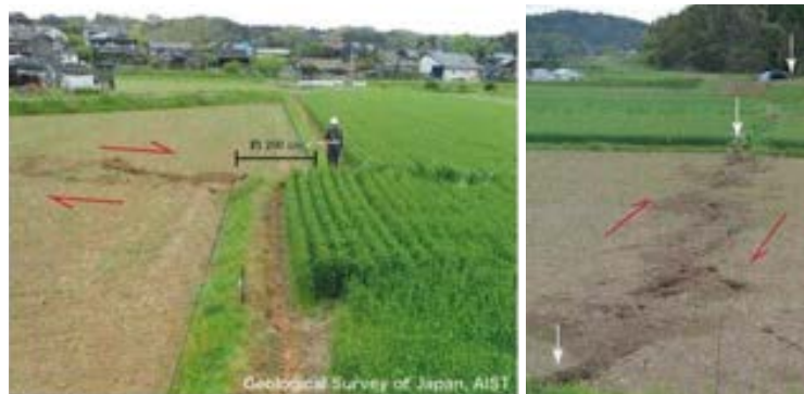
Fig.6 Earthquake surface fault along Futagawa Fault → Right lateral slip movement was observed
